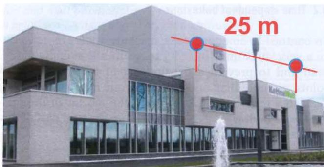
*Fig. 2. Building without movement joints; no visible cracks*
