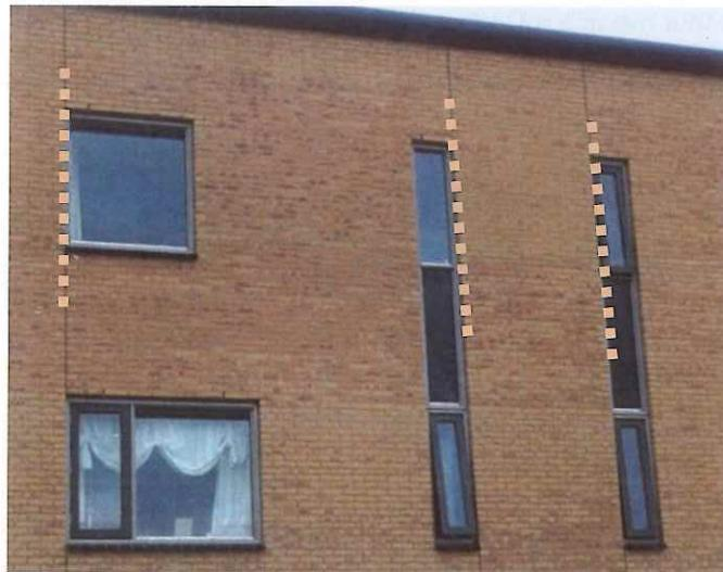
*Fig. 1. Building with small spacing of movement joints*
